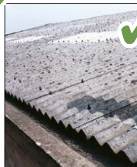
Asbestos cement roofing
